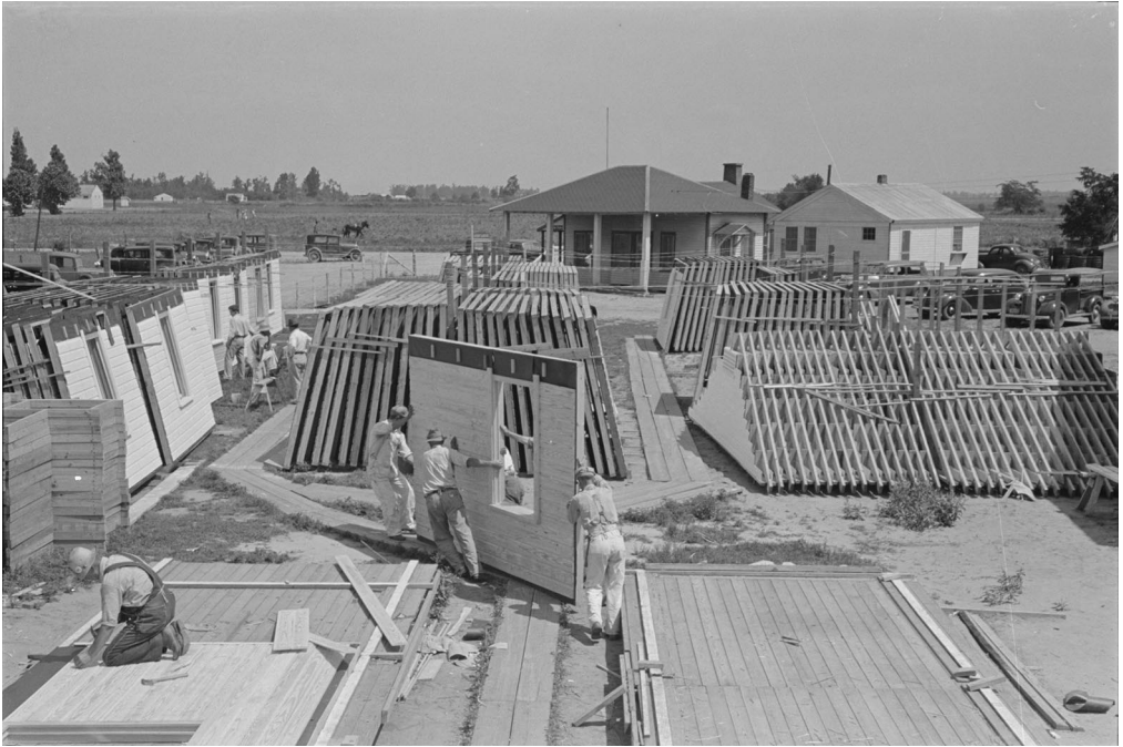
Figure 5. Type B and C Farmhouses, LaForge Missouri. 1933, FSA. Prefab Yard showing wall panels and roof trusses. Southeast Missouri Farms
