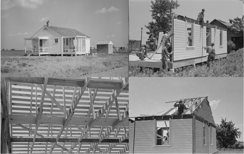
Figure 7. Type B Farmhouse, New Madrid County, Mo. 1933, FSA. Completed house, gable end and rafter setting, wall panels setting, skip sheathing
