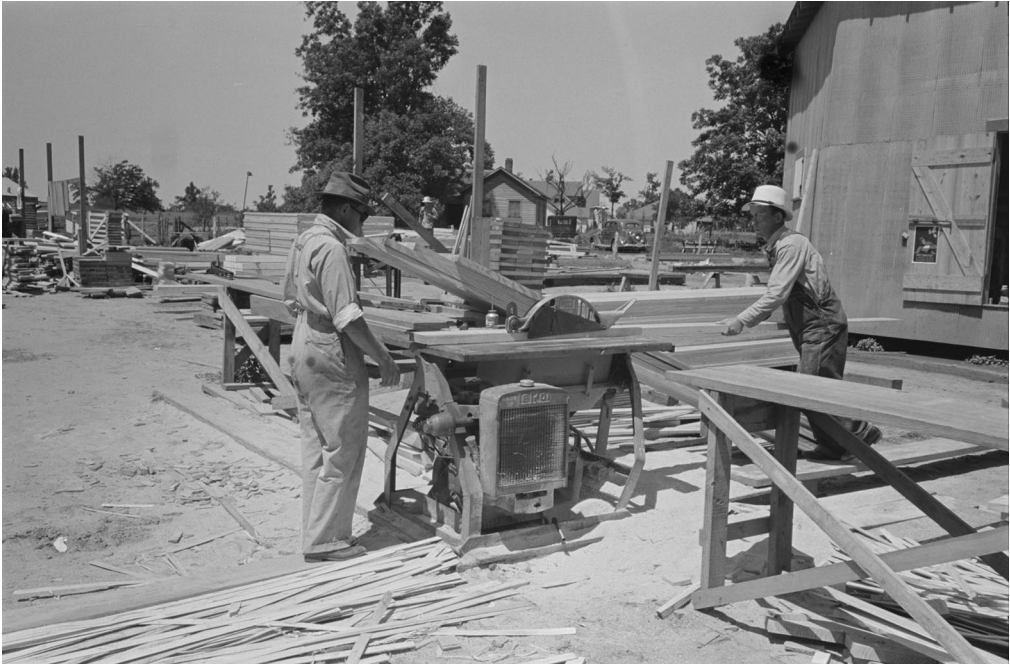
Figure 4. Type B and C Farmhouses, LaForge Missouri, Mo. 1933, FSA. Cutoff saw and guard at prefab plant
