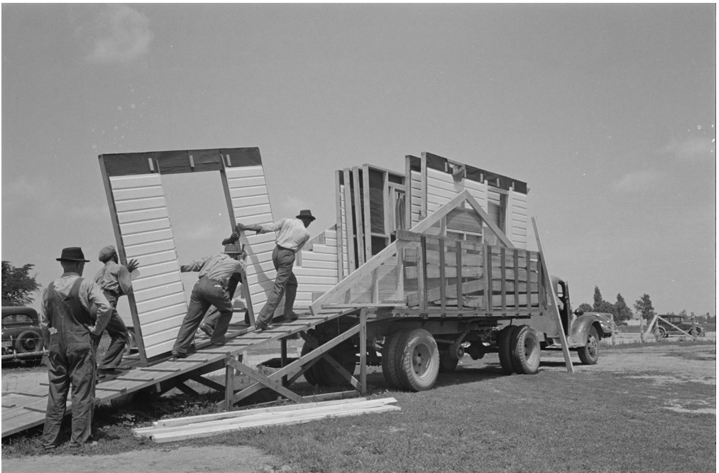
Figure 6. Type B Farmhouse, LaForge Missouri. 1933, FSA. Loading wall panels toaster style
