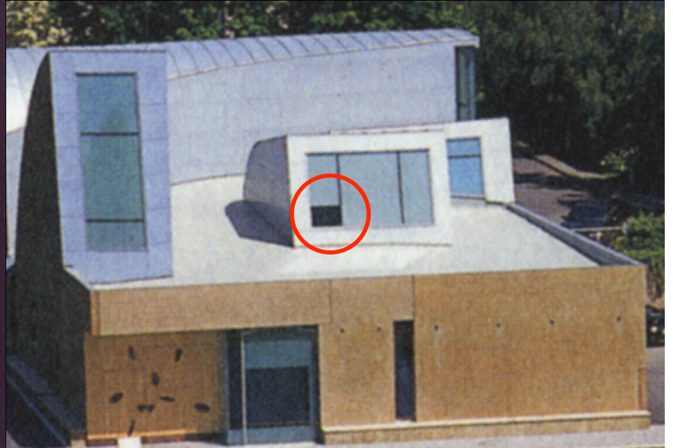
Narthex: South light, green lens, red reflector
