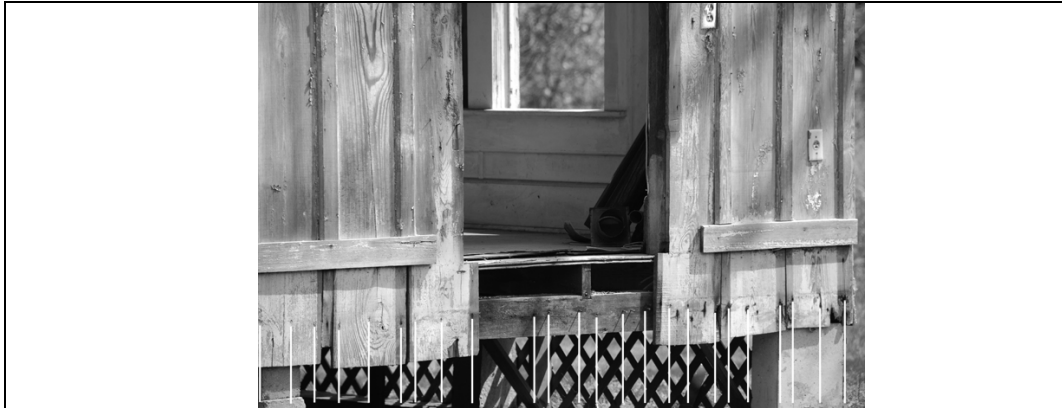
Figure 3: Joseph V. Frnka historic site, photo of vertical load bearing wall-board with 8 penny nails, reference lines at bottom indicate observed nail locations.
