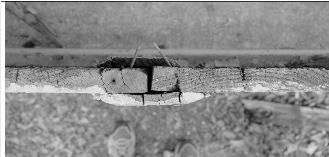
Figure 2: Interior and exterior batten strips over joints in one by wall boards, Joseph V. Frnka house, Front and Water streets, Columbus, TX.
